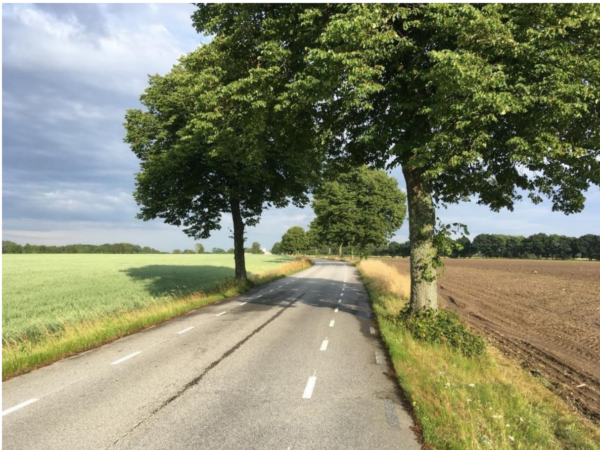
Figure 13: 2-1 road in Sweden with a central, shared lane for both traffic directions. (Source: © UFO-monumentet, https://commons.wikimedia.org/wiki/File:Bygdev%C3%A4g.jpg license: https://creativecommons.org/licenses/by-sa/4.0/deed.en ; No modifications)
